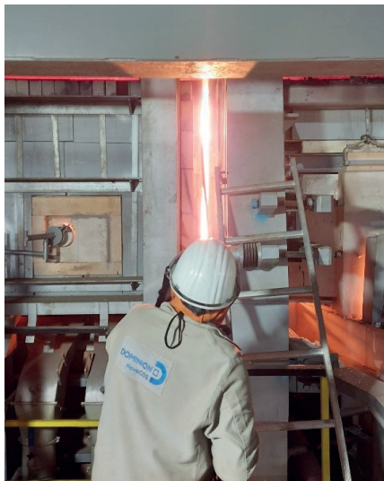
▲ Pic 4. Sealing external joints after heating-up a furnace.
