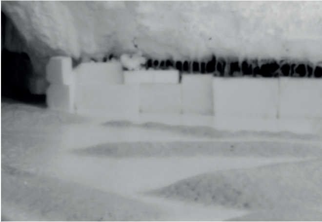
▲ Pic 5a / 5b. Repair of tuck stone area close to doghouse, before (5a) and after (5b) ceramic welding.
